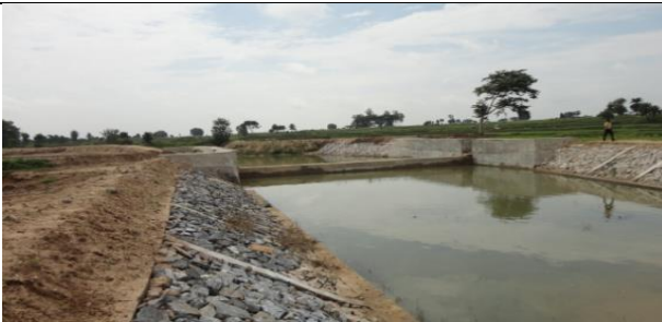
Check Dam at Mouza-Kolakata-Chepra, Block-Purulia-II
