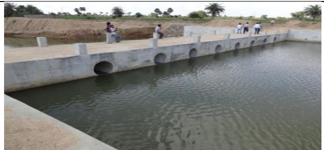
Check Dam cum Causeway at Mouza-Alkusha, Block-Para
