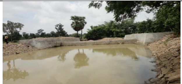
Check Dam at Mouza- Sindurpur-Chunardih Block- Purulia-II
