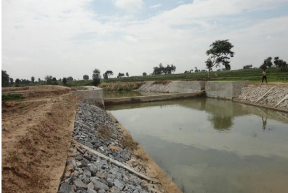
View of a typical check dam under RKVY within District : Purulia
