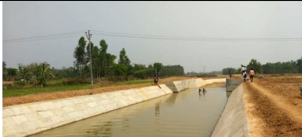
Check dam over Baghajole khal at Baghajole, block: Joypor, Dist : Bankura
